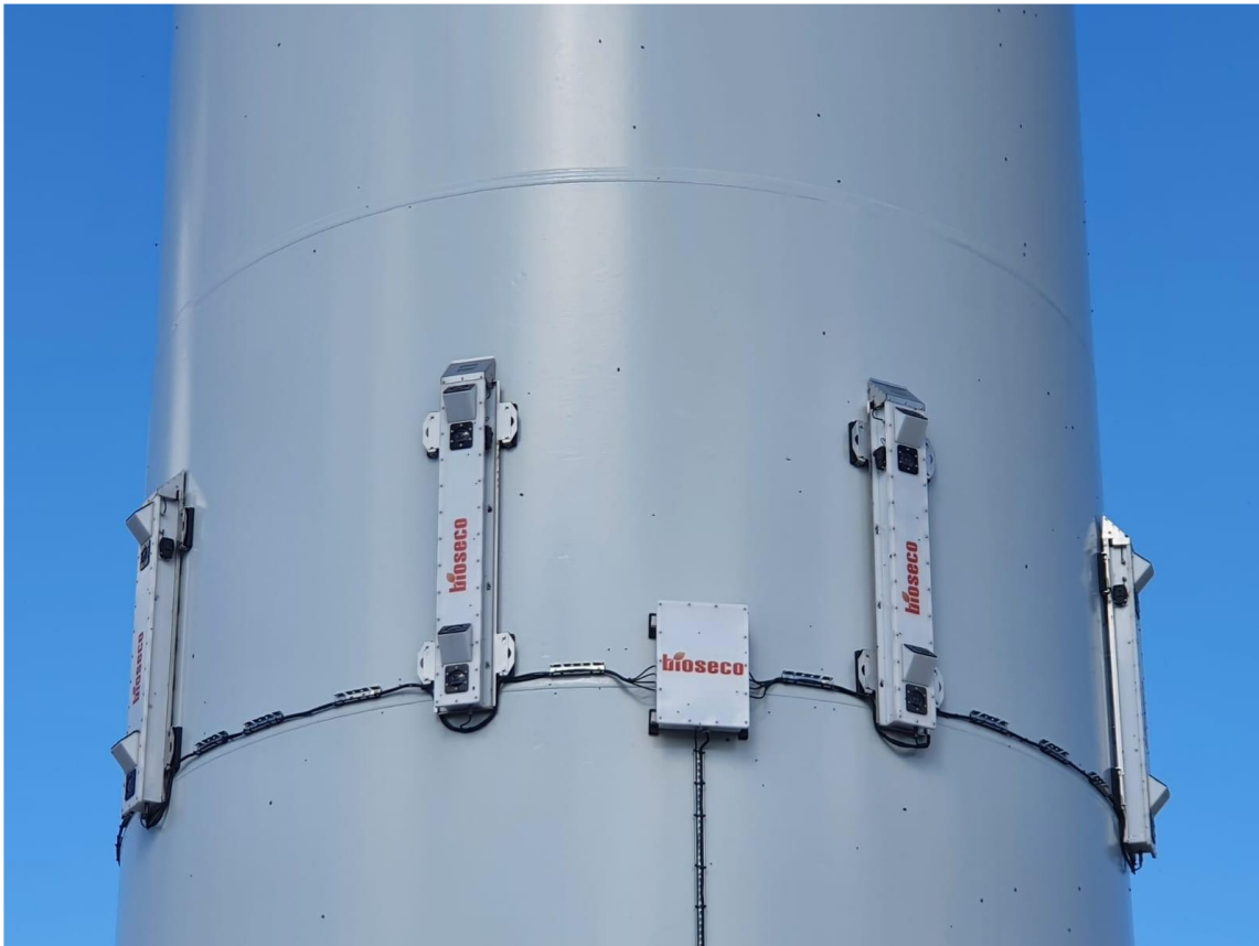
Fig. 2.4: Detailed view of the individual Bioseco detection modules (photo: BioConsult SH 2022).
