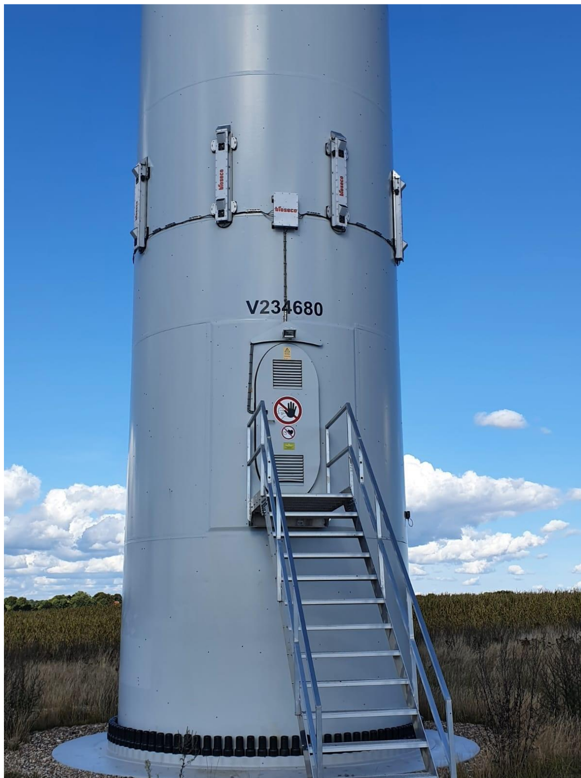
Fig. 2.3: The Vestas WT in Lentförden with eight Bioseco systems installed at a height of 7 m (photo: BioConsult SH 2022).
